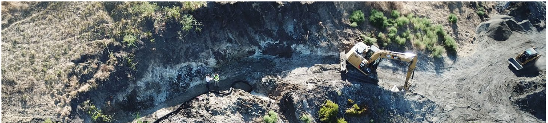
Example of geologic mitigation and repair work
