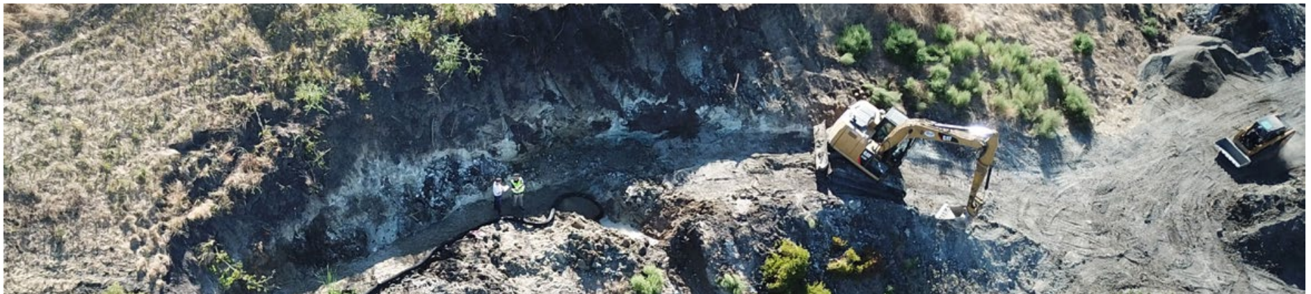
Example of geologic mitigation and repair work
