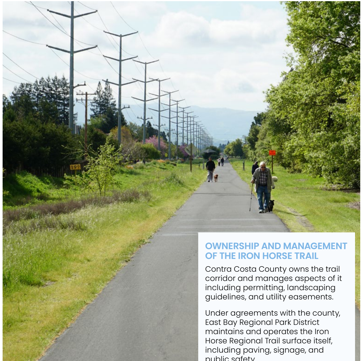
IRON HORSE TRAIL LOOKING SOUTH TOWARD DUBLIN
